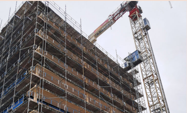
Construction Progress | ETC Bygg
