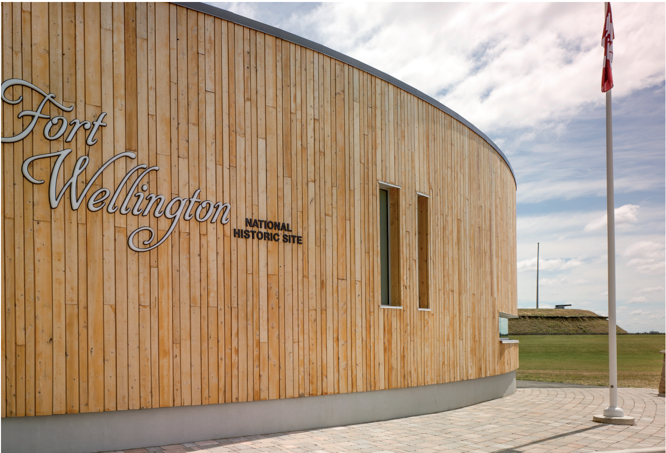
Wood Cladding at the Fort Wellington Visitor Reception Centre | DIALOG
