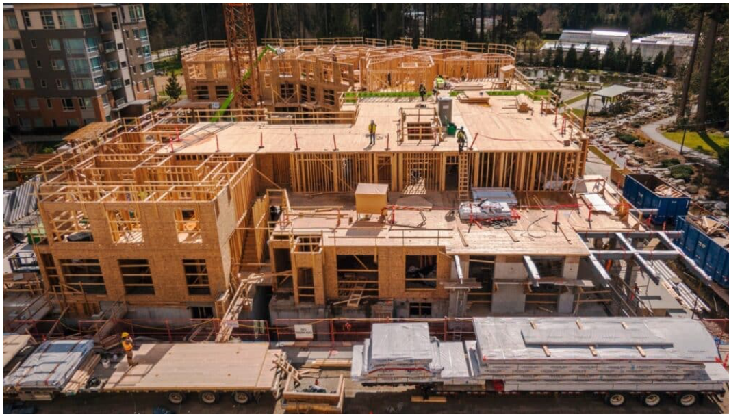
Figure 6. The combination of CLT floors with wood frame walls is an efficient form of construction for multifamily residential buildings (photo credit: Pollux Chung, Seagate Structures, courtesy naturallywood).
