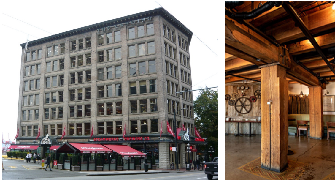
Figure 1. The Kelly Douglas building at 375 Water Street, Vancouver (now known as The Landing) is a nine-storey heavy timber structure that was built in 1905 (source Wikimedia Commons).
